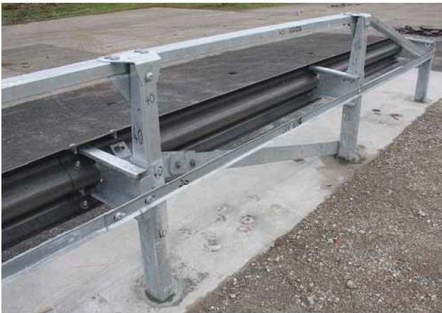
Tirant entre les supports n°40 et 41 / ↑ Brace between posts nrs. 40 and 41 / Tirante tra i paletti n°40 e 41
